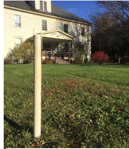
Figure C14. The falling head infiltration test in progress at the School Street apartment site.
