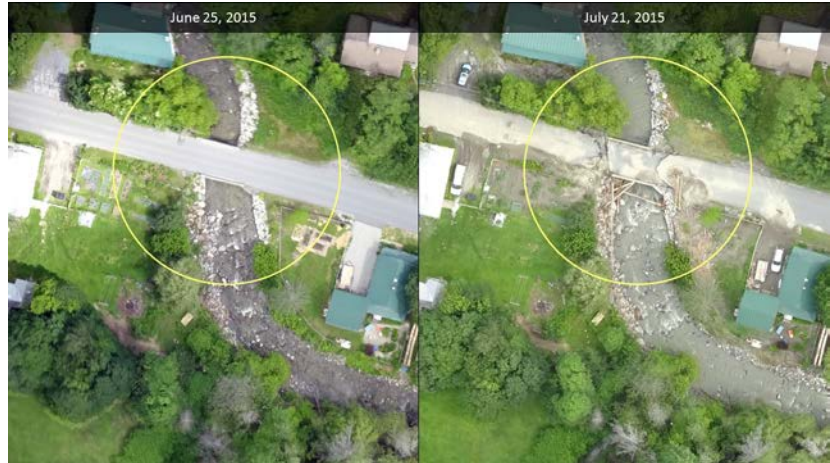
Figure C2. Flooding-related damage in Great Brook following a high intensity rain event. Imagery collected by the University of Vermont Spatial Analysis Lab (2015).
