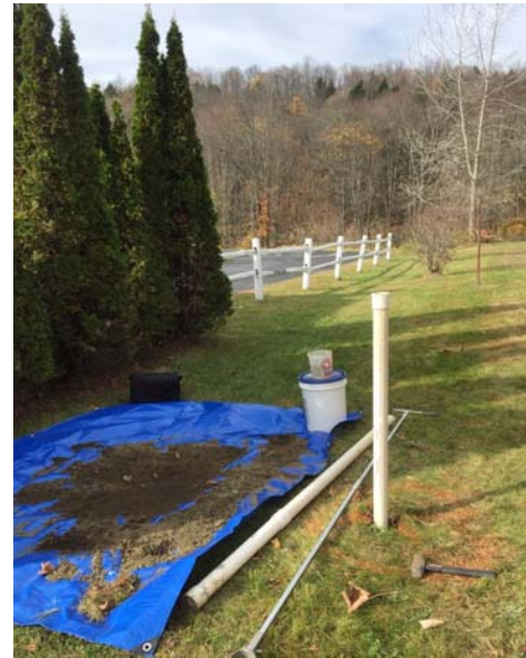
Figure B16. Infiltration testing using the falling head method in progress at the Wilkins Harley-Davidson site.
