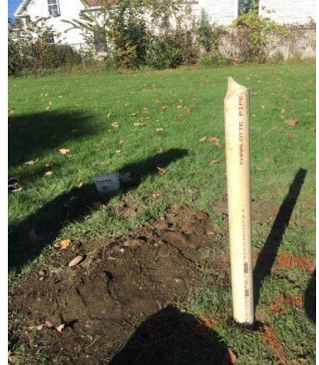
Figure A14. An example of the Falling-Head Borehole Test in progress.
