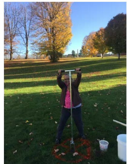
Figure A16. CVRPC staff assisting with soils testing in the grassy area along Washington Street where the proposed infiltration practice would be located.
