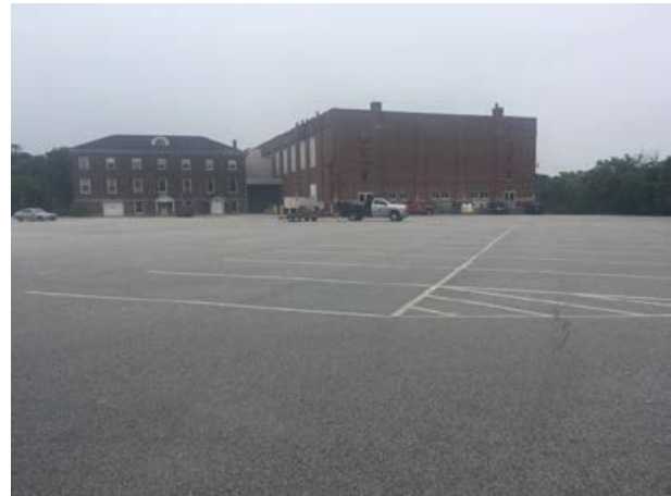
Figure A11. The subsurface sand filter is proposed under the auditorium's large parking lot.
